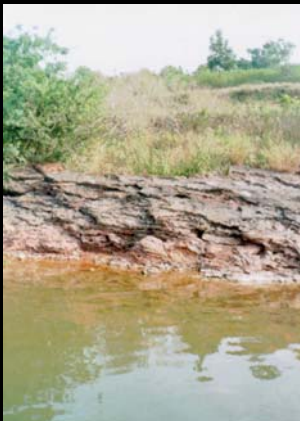
Erosion from weathered rocks
