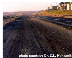
Figure 2.23: Completed CTB with Curing Sediment Figure 2.24: Lean Concrete Base Material
