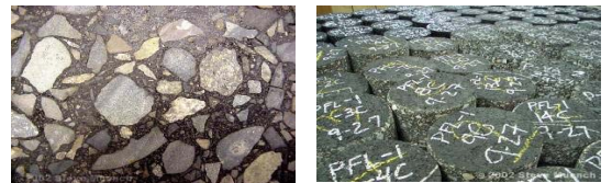
Figure 4: Dense-Graded HMA Figure 5: Dense-Graded Cores
