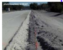
Figure 3: Limerock Base Course Undergoing Final Grading
